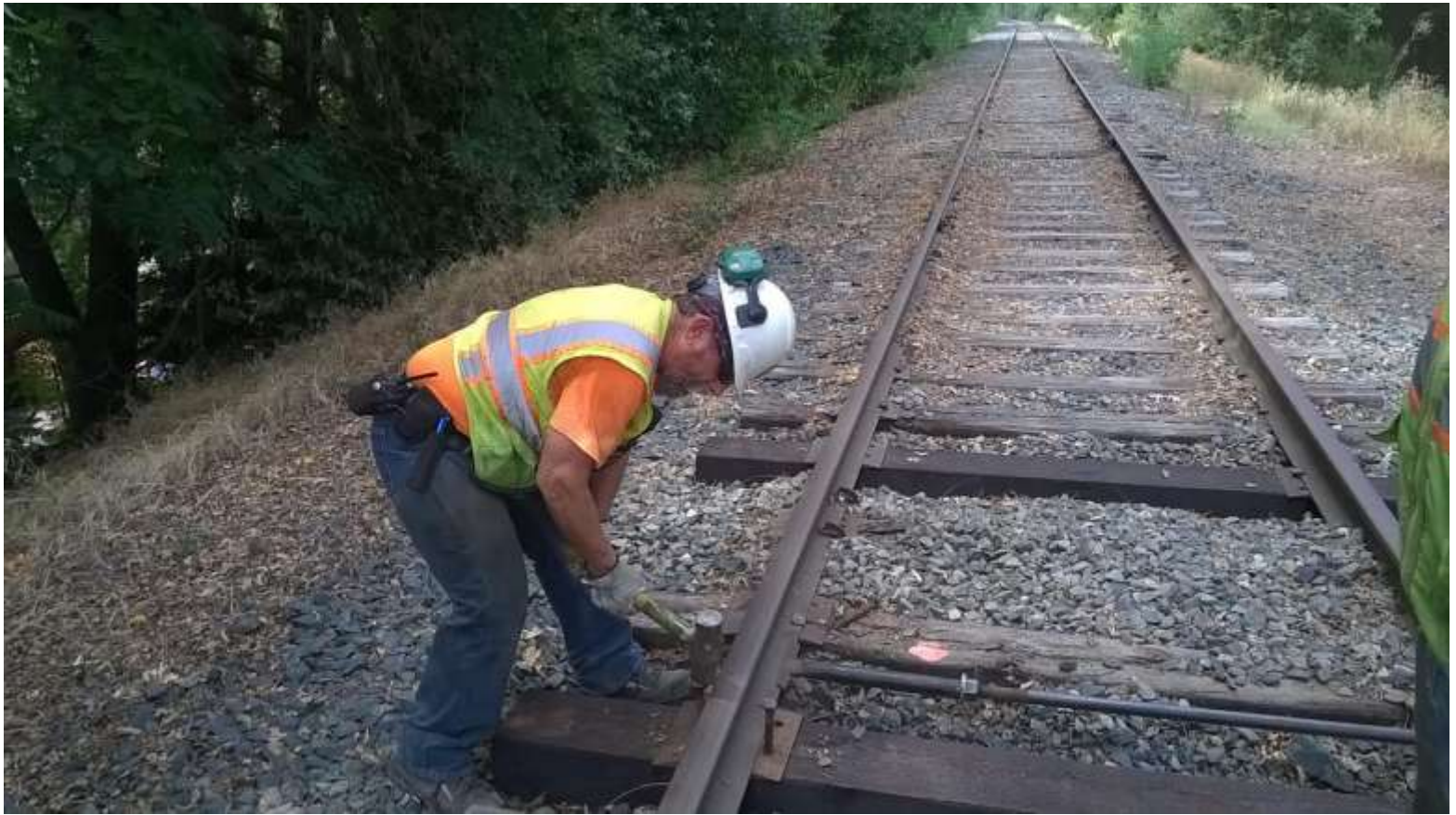
Joe sets spikes after the rail-spreader was used to re-gauge the track
