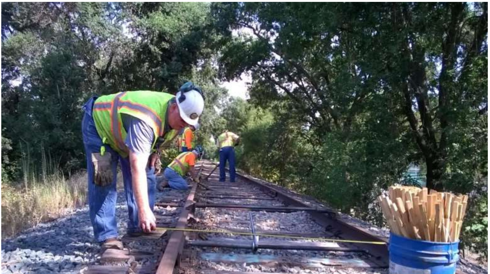
Chris checks the gauge after having employed the use of the rail-spreader
