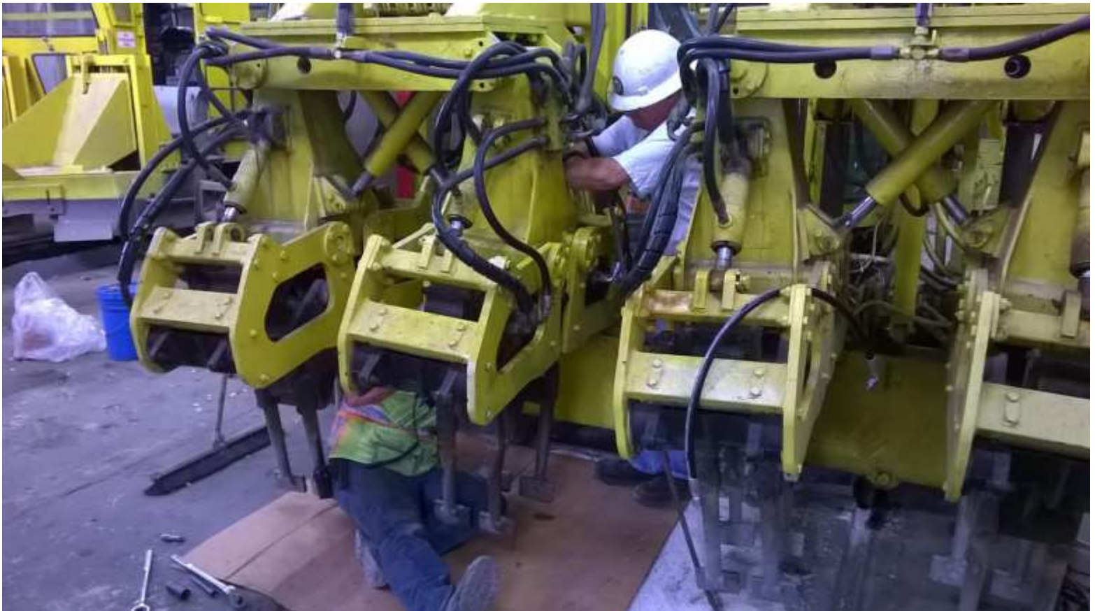
Joe and Mike H. hook up the tamper's new hydraulic hoses
