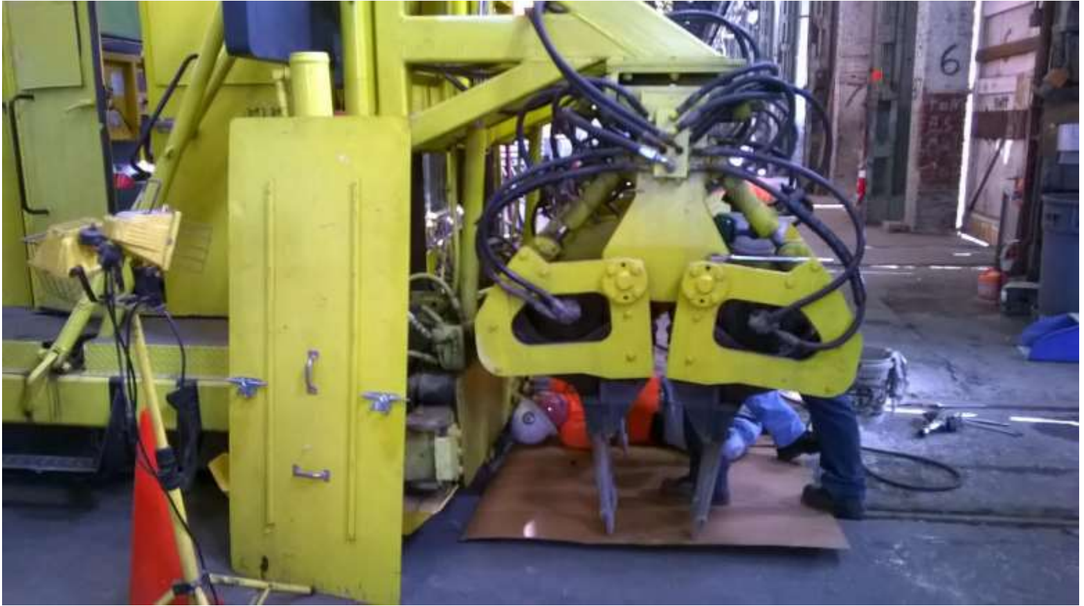
Mike H. lying down on the job – in order to access the tamper's vibrator motor, of course...
