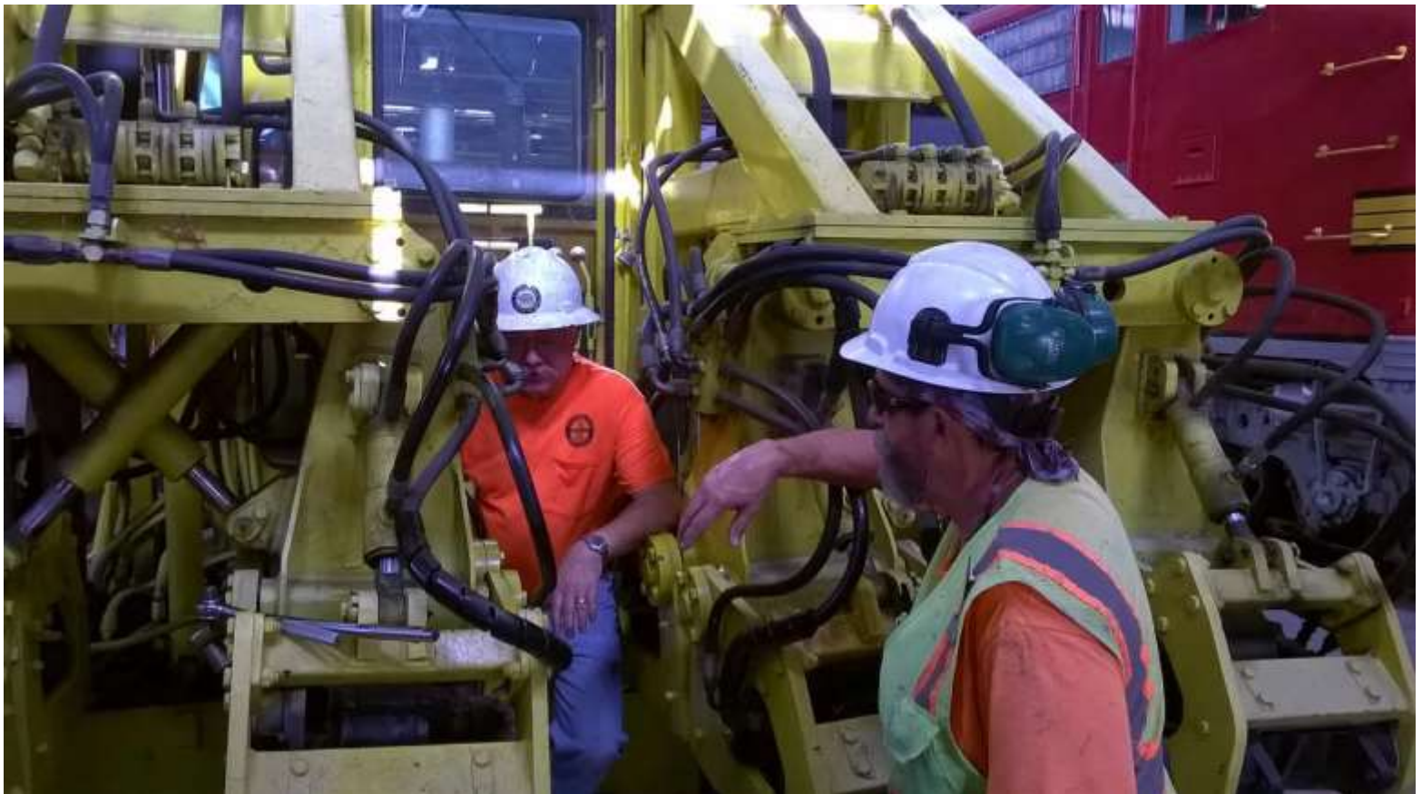
Mike H. and Joe assess the problem with one of the tamper's vibrator motors
